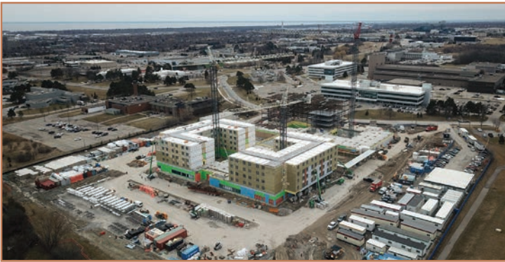
March 2022: Northwest view of the project with the modular installation in the foreground. Structural steel erection and Speakman Drive in the background
