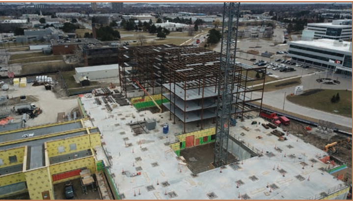
March 2022: Southernly view of the West Building's structural steel and the second level concrete deck
