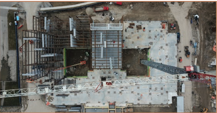
March 2022: Aerial view of the West Building's structural steel erection and second level concrete deck installation.
