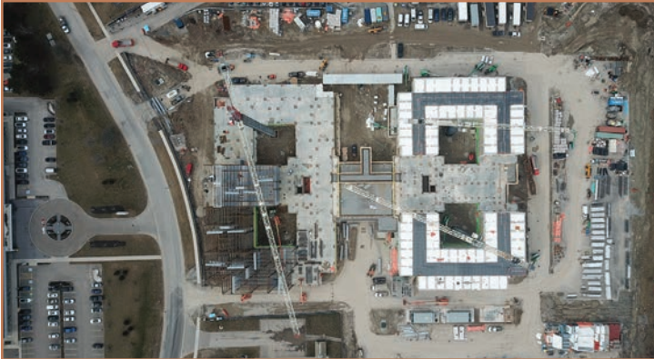
March 2022: Aerial view of the project with structural erection on the west (left) building and the modular installation on the east building.
